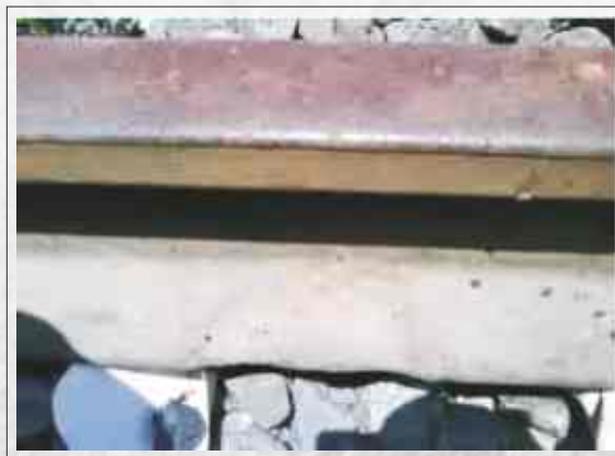
Corrosion of rails in the liner region
