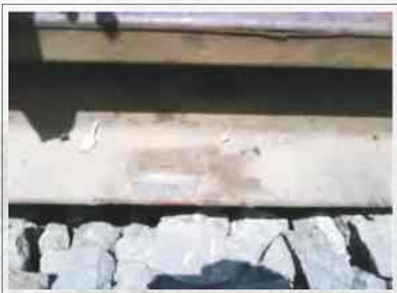
Corrosion of rails in the liner region
