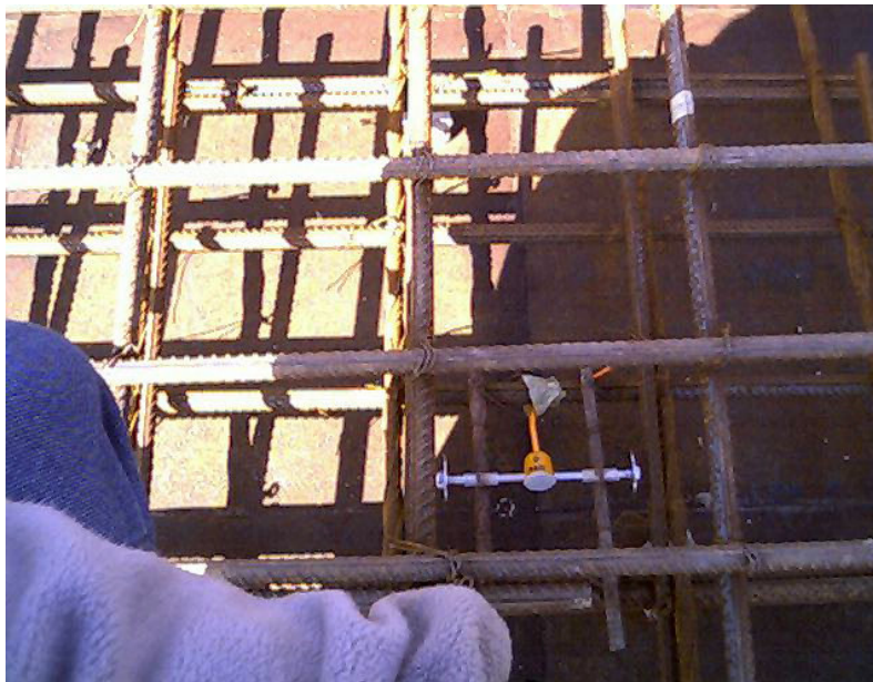
Figure 11. Installation of VW strain gauge
