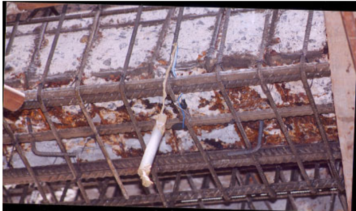
Figure 4. Embedded sensor in beam.
