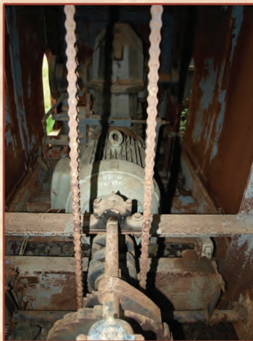
Drive unit assembly for Radial Gates
