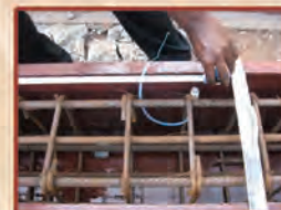
Chloride sensor in RCC beam exposed to naturally corroding condition at NIT, Suratkal
