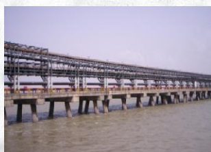
Corrosion monitoring of port structures
