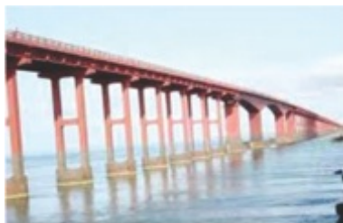
Pamban bridge is coated with this multicoat system
