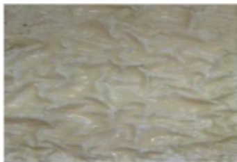
400 \mu coating lifted from the steel surface after 2 Hrs
