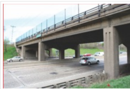
Corrosion free concrete structure
