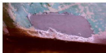
De-rusted coach portion
