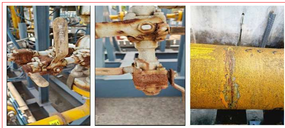
Figure 1. Images of the coatings applied on CNG pipeline terminals at Taloja CGS terminals of MGL.
