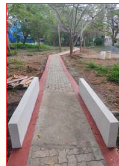
Figure 3. Demo pedestrian pathway using sustainable paver blocks.
