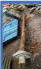
Fig. 2 Excavated mild steel anode
