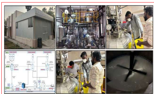
Figure 1. Installation and commissioning of pilot plant (10 kg/batch) at CECRI site.
